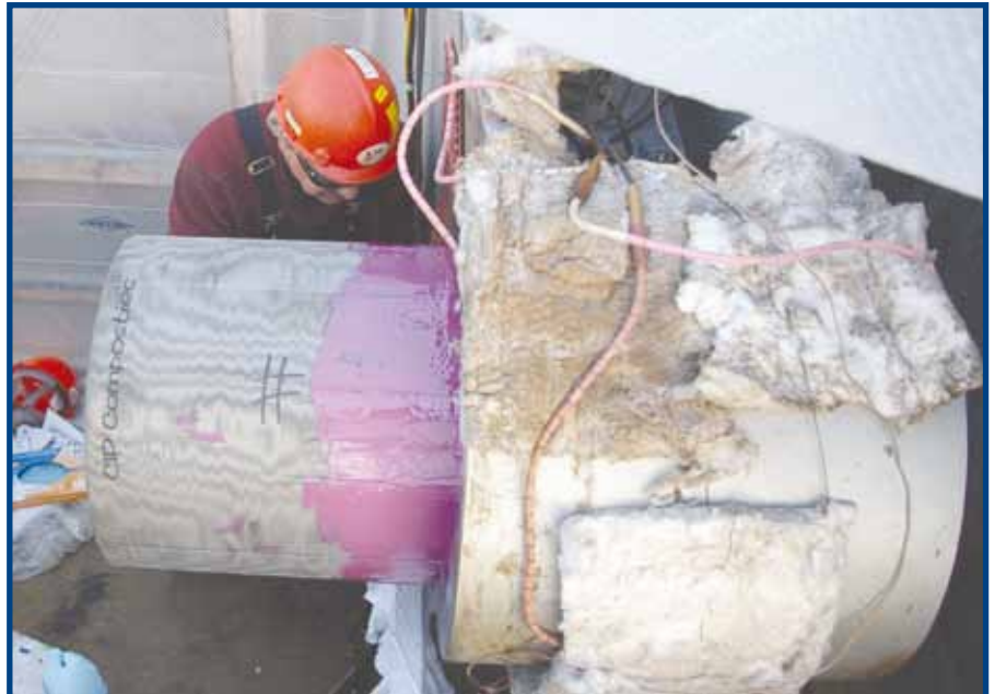
RADIAL SPILLWAY GATE TRUNNION BUSHINGS
