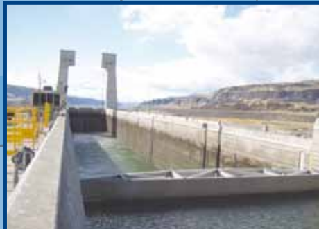
LOCK GATE - JOHN DAY DAM
