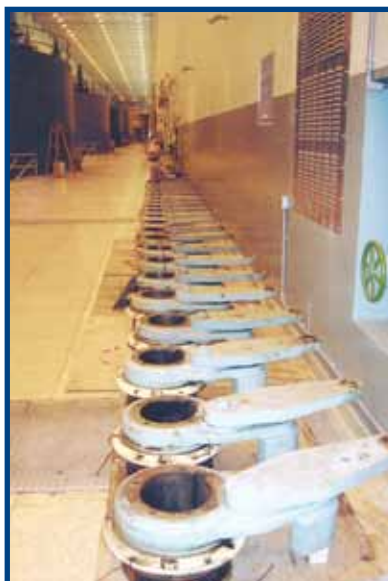
WICKET GATE READY FOR REBUILD
